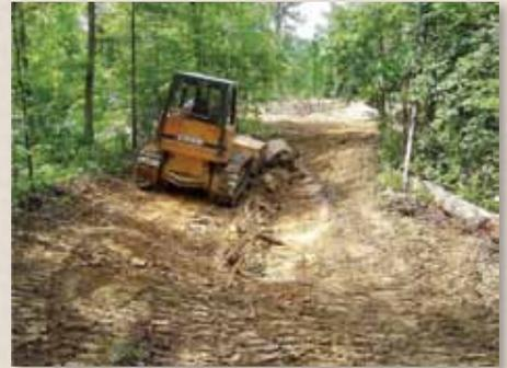
12. Use a construction level to check the depth of the depression. In locations east of the Mississippi River, the wetland can be expected to contain water year round if it is built 18 inches or deeper. If it is shallower than 18 inches, it may only contain water seasonally.
