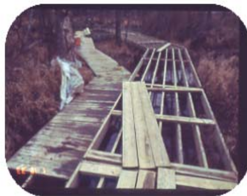
Upgrading an Existing Boardwalk
